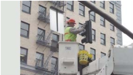
A City-bired contractor installs one of more than 13,000 LED lamps during the fall of 2001.
