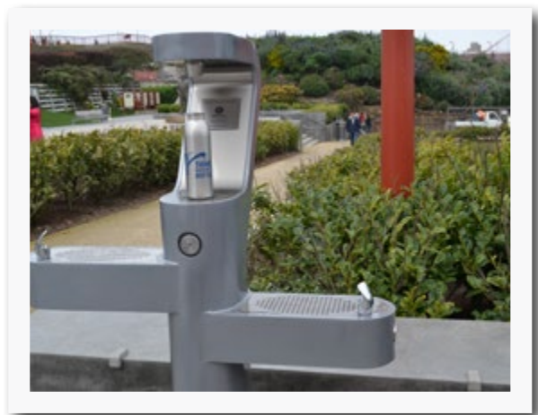
This water refill station at Golden Gate National Recreation Area is one of many infrastructure options for parks to consider.
